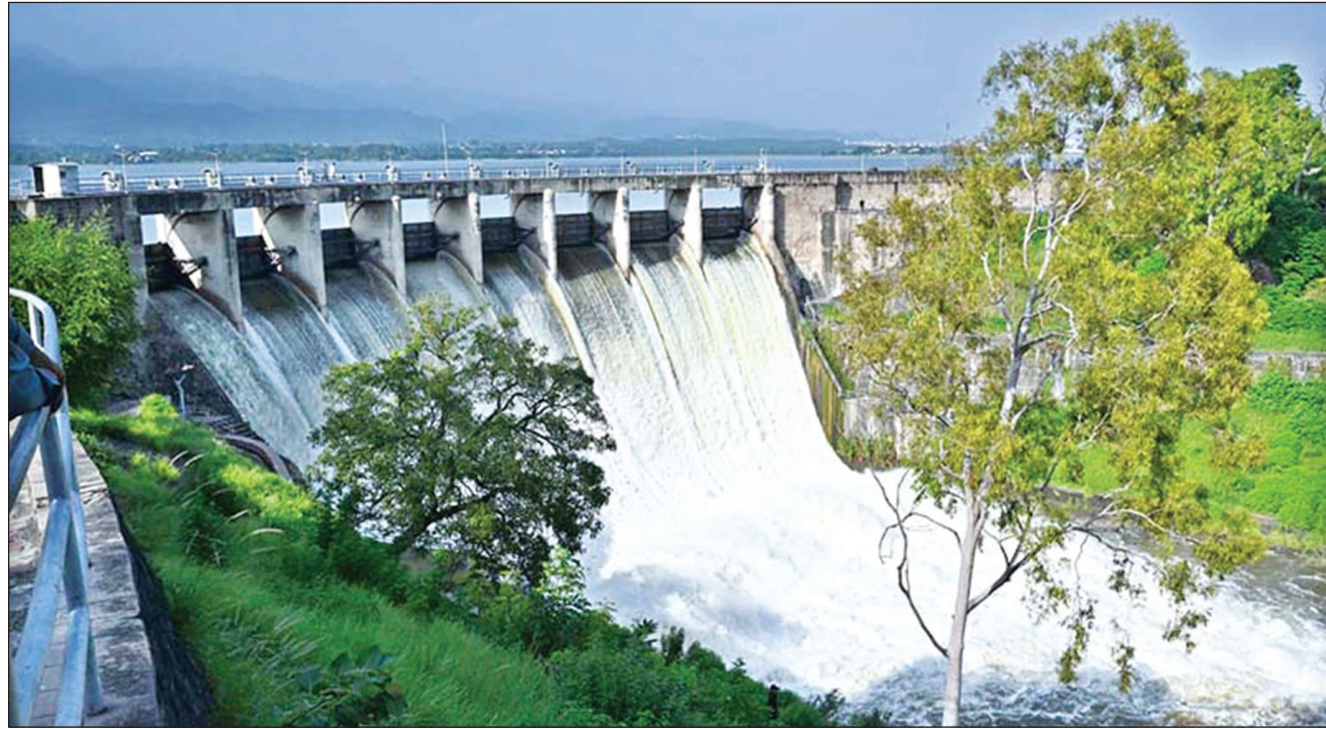
ISLAMABAD: Rawal Dam authorities open spillway of the reservoir after dam water level rose to alarming level due to heavy rain. APP
